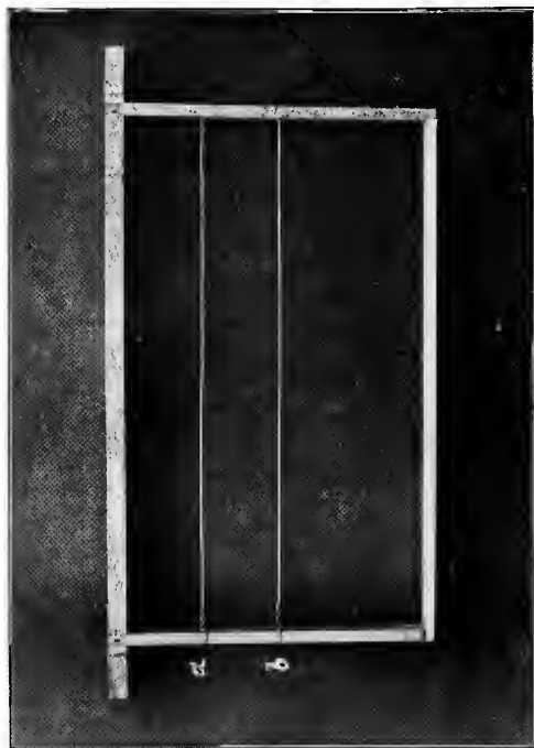
FIG. 23.—WIRED FRAME, a, b , Places where wire is tied to Frame.
