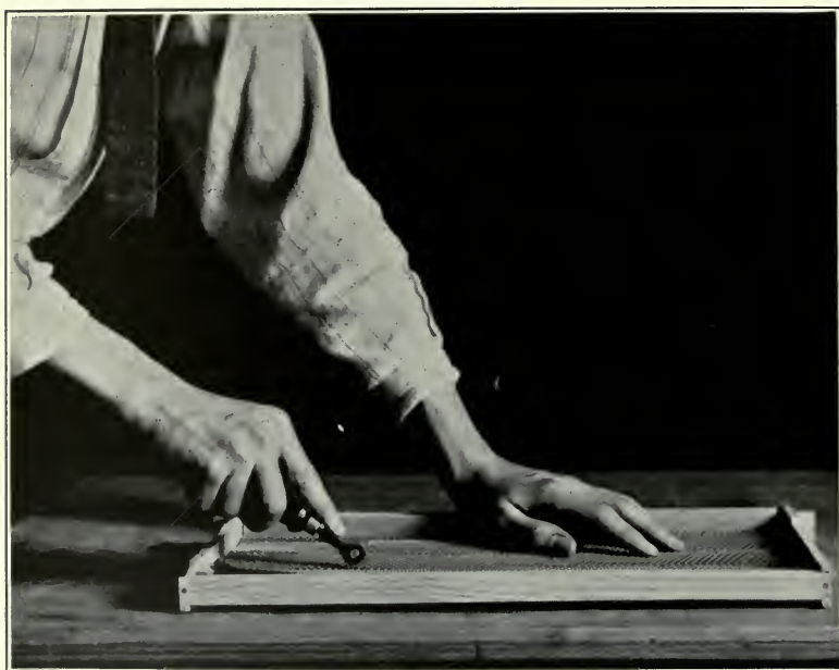
Fig. 19. Embedding Wire in Foundation.
